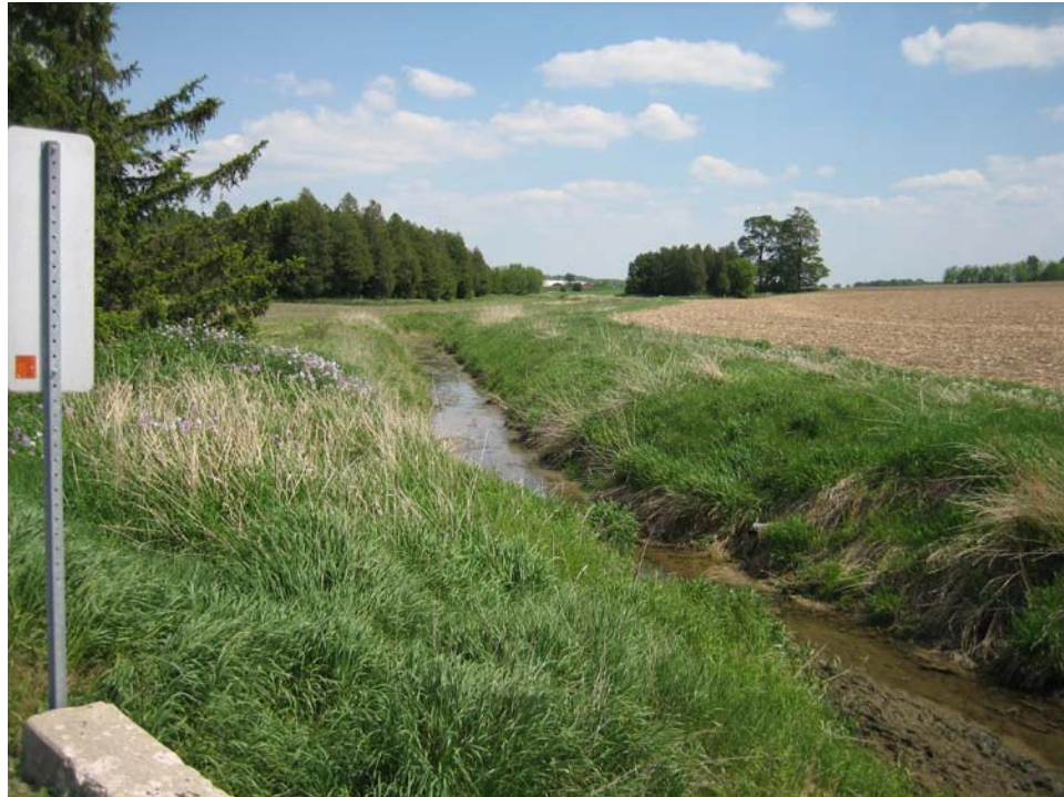
13. Cox Creek looking downstream from Kenning Place. All flow is from tile drains.
