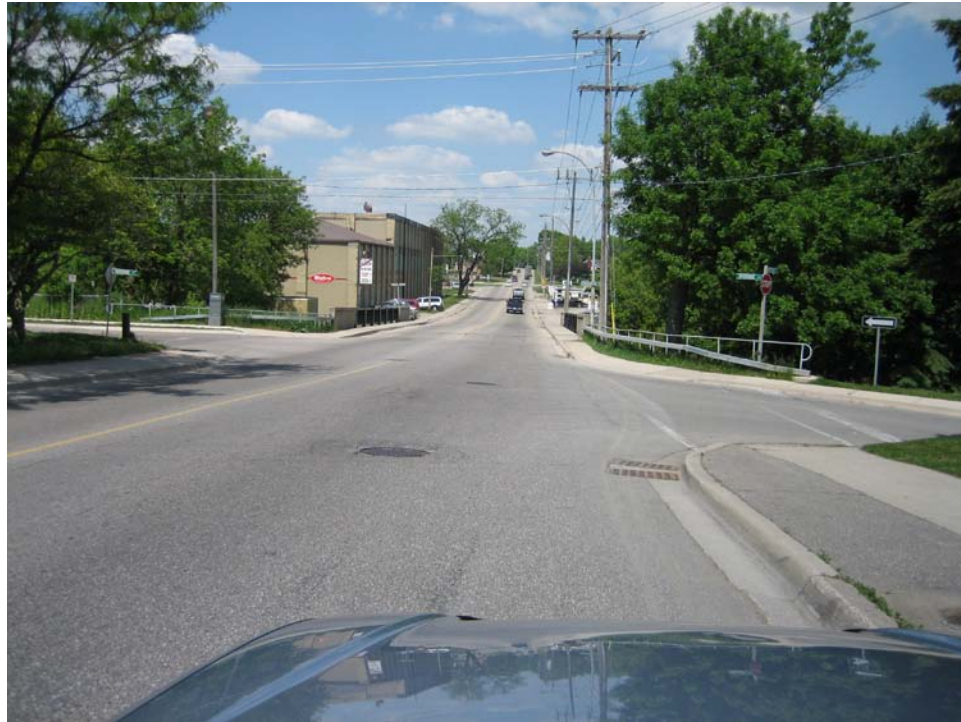
1. Canagagigue Creek crossing looking north on Arthur Street.
