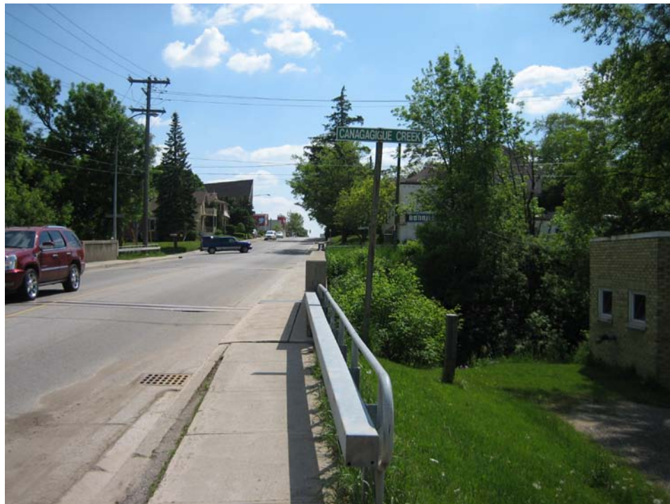
2. Canagagigue Creek crossing looking south on Arthur Street.
