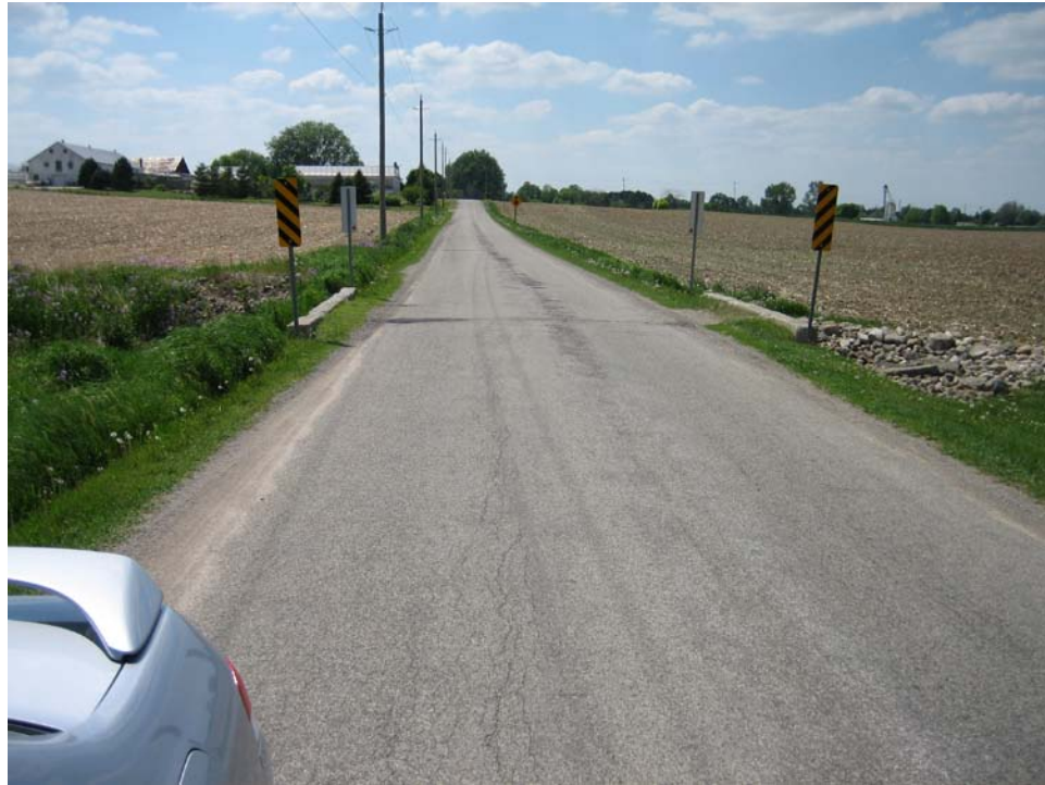
11. Cox Creek crossing at Kenning Place.
