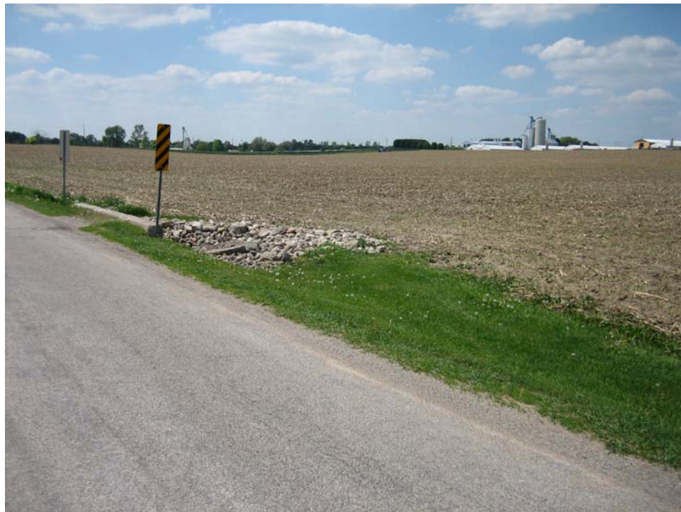
12. Cox Creek alignment looking upstream from Kenning Place.
