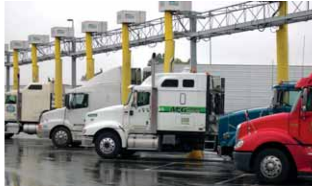
Trucks parked at New York Thruway rest area shut off their engines and plug into IdleAire facility for heat and electricity.
